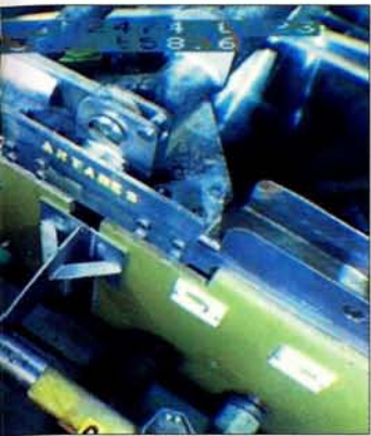
er connection to the junction e of Nautil's manipulator arms in the interlink cable, while the ble) grips the "ballet rail".
